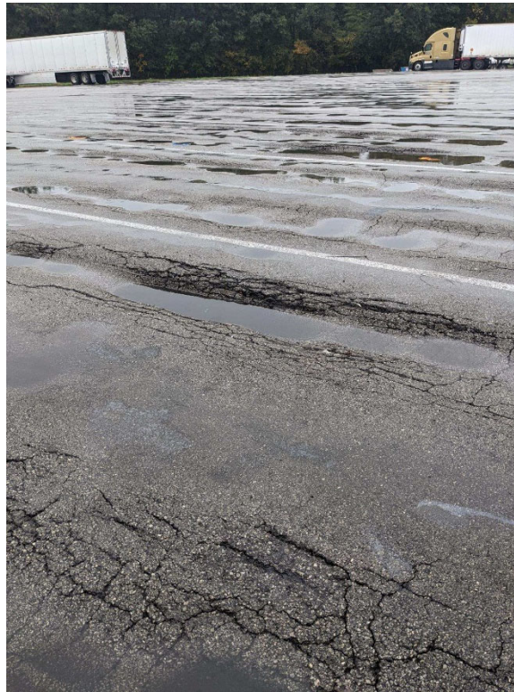
Figure 2. Typical pavement condition in westbound truck parking plaza (north side of ITR).
